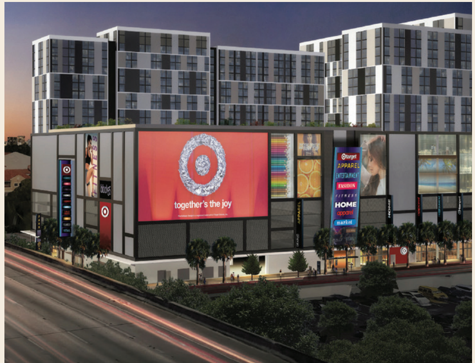
Sawyer's Landing is a 578-unit affordable housing project with Target-anchored retail in Miami's Overtown.
